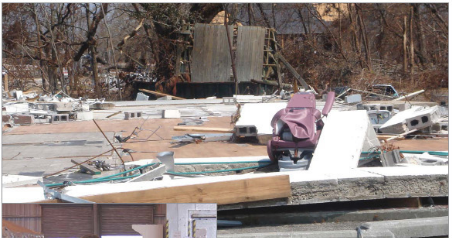
A dental office destroyed by Hurricane Katrina.
